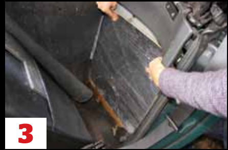
3 Trial fit each piece of barrier mat, making sure it doesn't cover any of the 10mm securing bolts for the firewall panel (trim the edges if necessary). When fitting each piece, use your fingers to mould it into the shape of the firewall panel.
