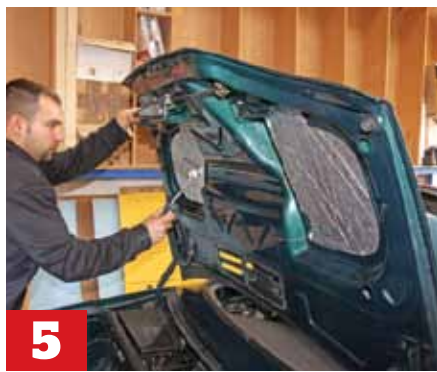
5 As ever, make sure the edges of the Vibrasorb are firmly pushed in position - use your fingers or a trim tool to manipulate the edges. Run over each piece with a decorator's roller to ensure they are securely stuck to the boot lid.
