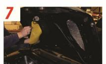
Another area of the boot to be soundproofed is the underside of the boot lid. The single skin areas can be covered in self-adhesive Vibrsorb, which helps to reduce panel vibration and absorb sounds.
